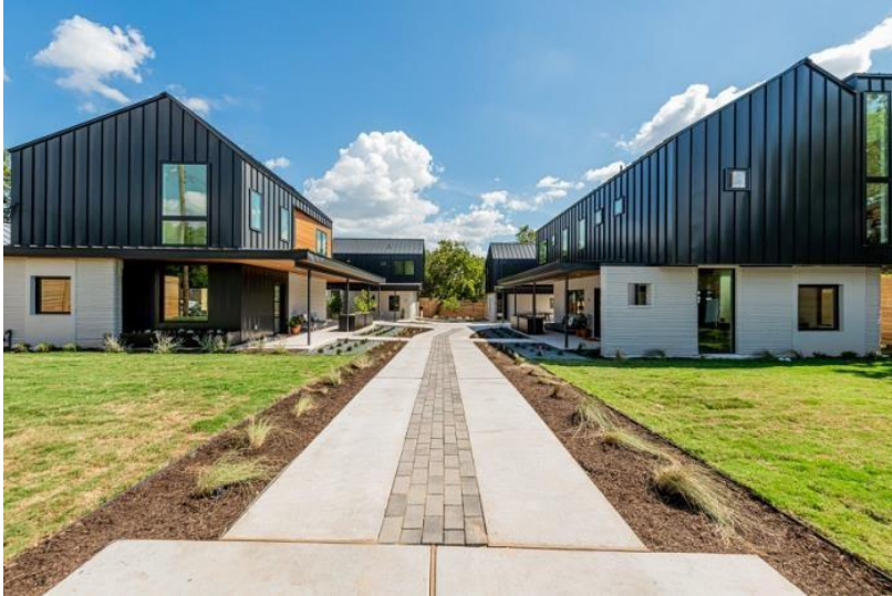
Pic. 5: General view of houses, ground floor created with 3DP in the USA.
