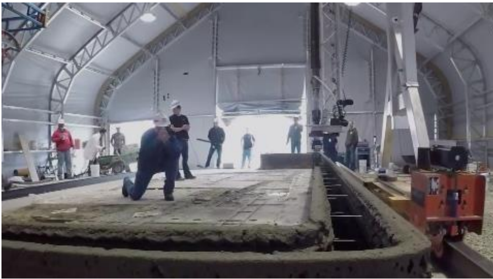
Pic. 7: 3D printing the new B-Hut. Photo by ERDC.
